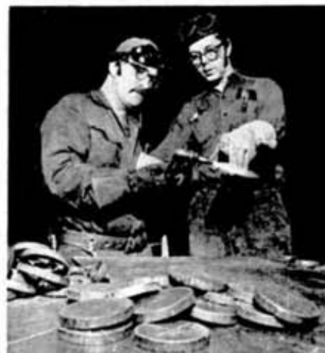
Surface operations play a vital role in the continuing operation and upkeep of underground equipment. Training is conducted in the surface shops as well, and Joe Brunet , left, an underground track boss, undertakes to learn the proper use of a cutting torch from plater Ed Black , of the Garson mine plate shop. Since the mine requires qualified burners to cut rails, bolts and fishplates, men are being trained to do the job by the experienced plate workers. Here Joe prepares to cut washers for the 4,000 foot level crusher at Garson mine.
