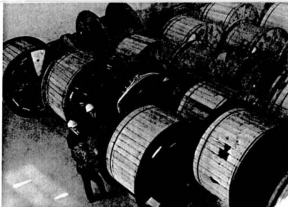
Hoisting rope plays a key role in the everyday activities of any underground mining operation and, at Inco, they transport approximately 9,000 people each day. At Frood mine's No. 3 shaft, a substantial amount of hoisting rope is kept on hand to replace cables in operation.
