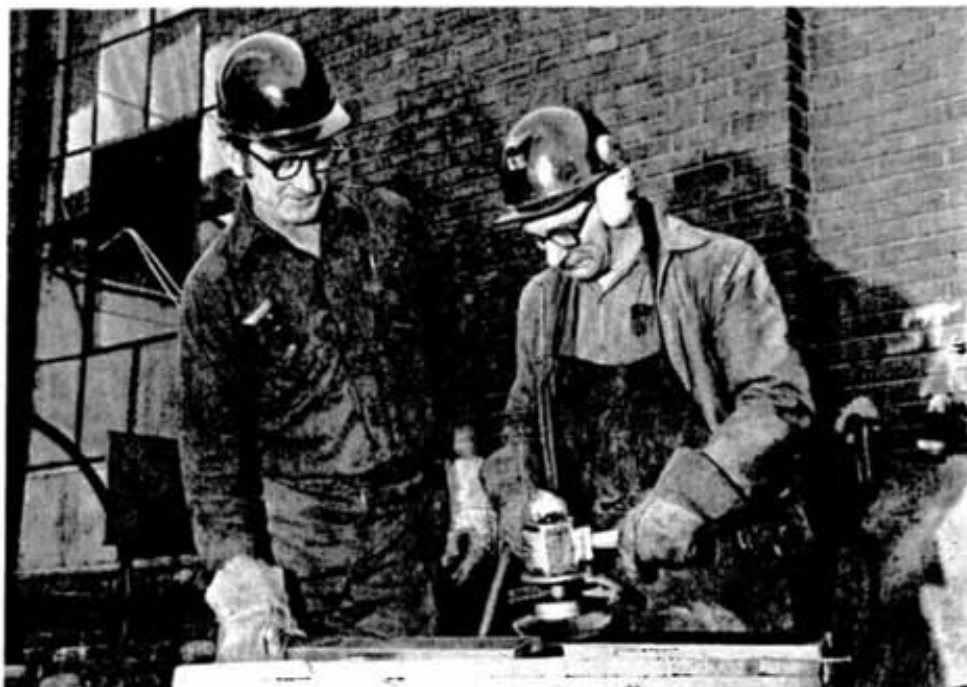
Clean equipment is reliable equipment, and reliable equipment is the only kind our riggers use. Here, Frood riggers Barney Sloan, left, and Raymond Bruneau, clean up a capel rope attachment before returning it to service. Each day, riggers examine, lubricate, and replace ropes when required.
