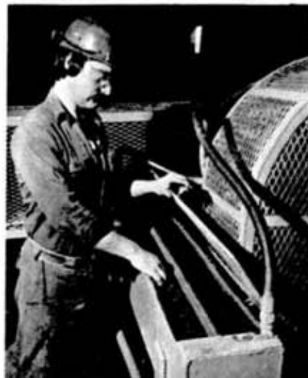
While the old method used in fluid drive cooling systems incorporated a copper tube with running water inside to cool the oil, maintenance crews at the Froid-Stobie mill have reversed the process and now use the water to surround the copper pipe containing the oil. This method of cooling pumps has now been applied to all the Froid-Stobie mill concentrate and tailings systems. Here Frank Boyd , a maintenance mechanic, inspects one of the newly installed units.
