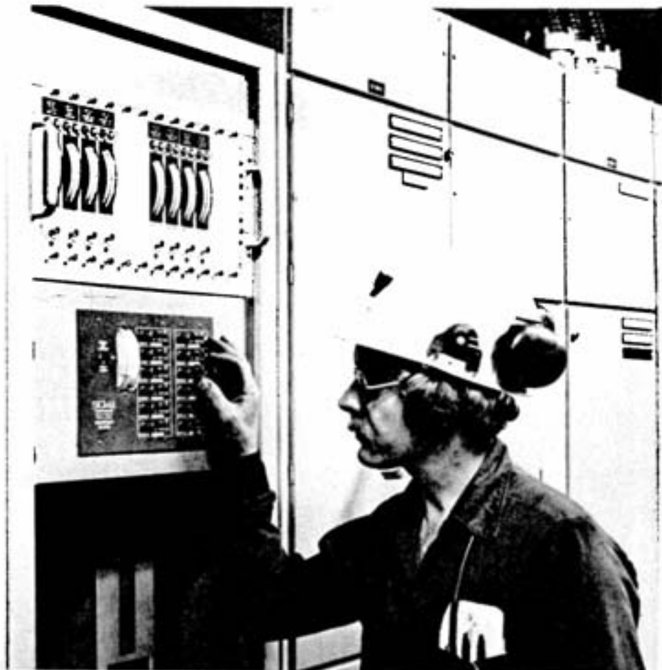
Eddie Peters, central maintenance foreman, checks the fan control monitoring centre. This centre picks up fan vibrations as well as bearing temperatures. Excessive readings will automatically shut down the fan and in turn set off an alarm on surface.
