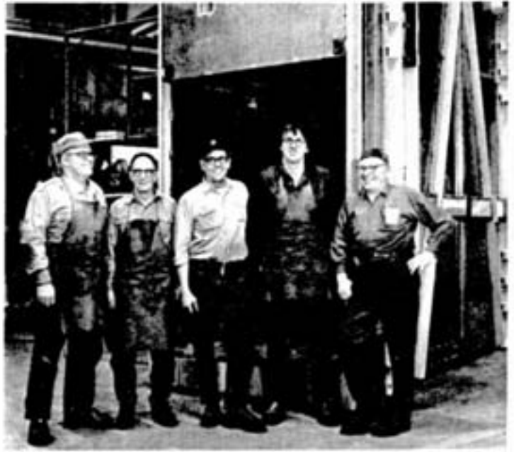
The divisional shops were responsible for constructing the new cage. Some of the men who worked on it are, from left, Mike O'Neill, Gerry Guerin, Walter Plante, Rick Preseau and John Muron
