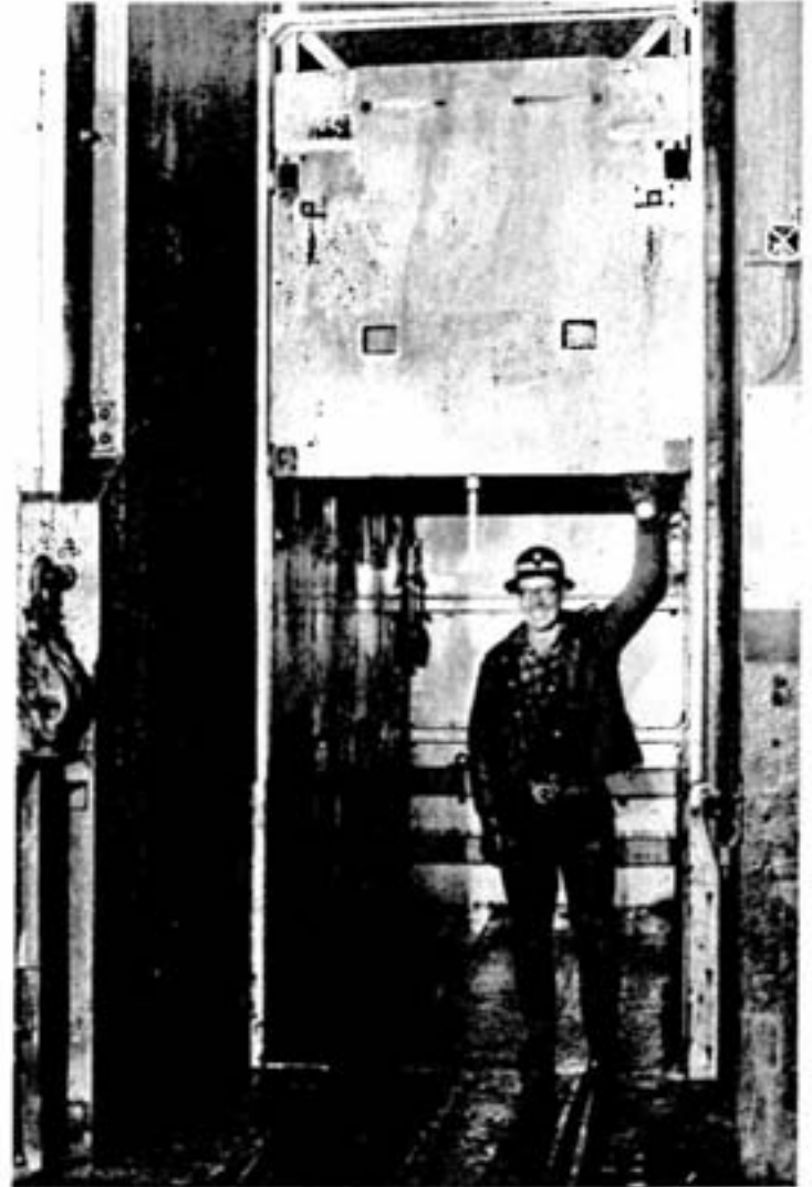
The new cage is now installed at Stobie seven shaft. Cage tender George Jolicoeur gets ready to "take her down".
