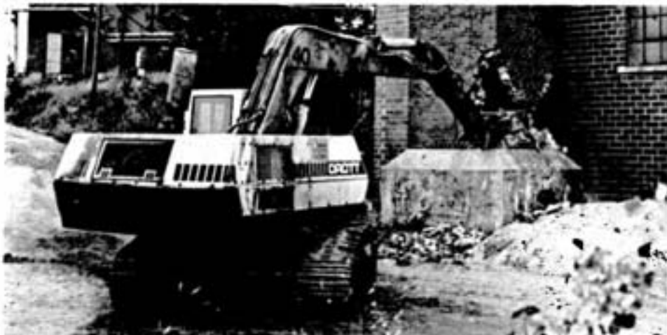
The crane buries its plunger into the base of the stack preparing it for the coup de grace.
