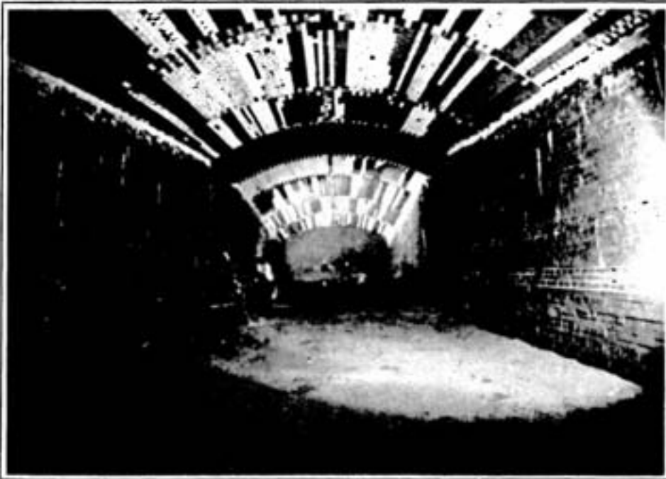
The interior of the copper flash furnace.
